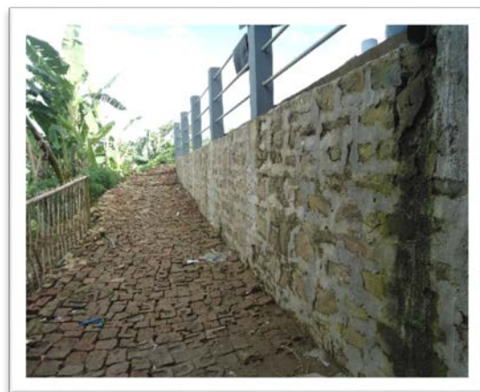
2 (two) Protection Walls
