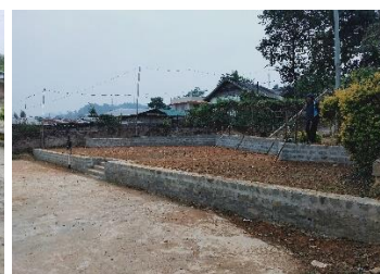
Retaining Walls for Mini-Park
