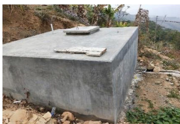
RCC Water Reservoir (10,000 L)
