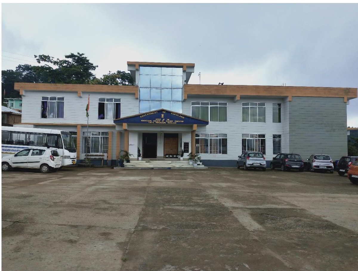
MCTE Academic cum Administrative Building
