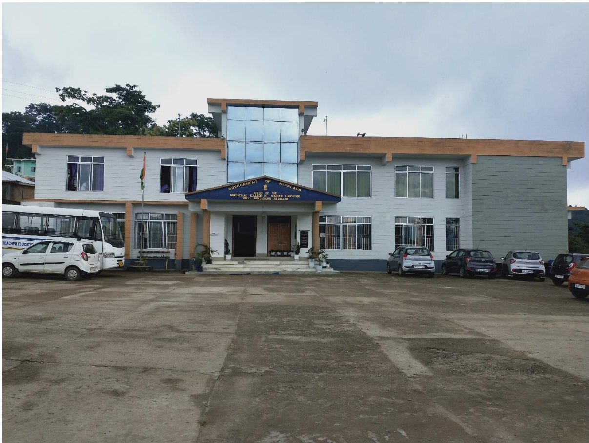
MCTE Academic cum Administrative Building
