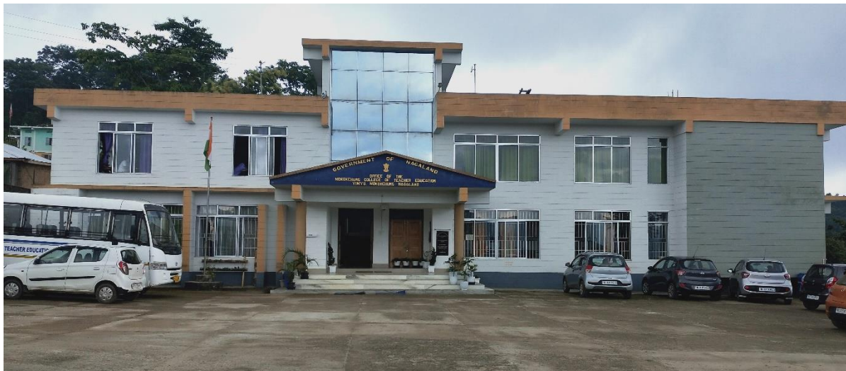
MCTE Academic cum Administrative Building
