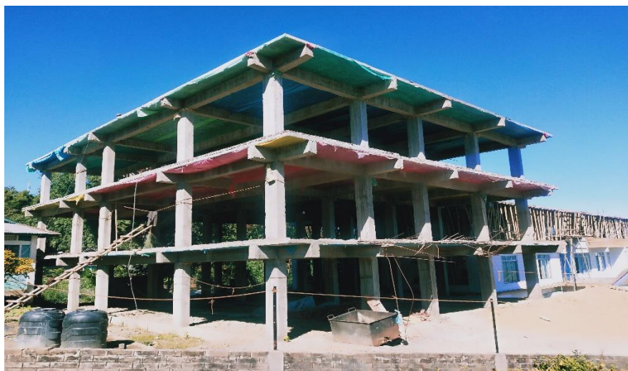
MCTE New Academic Building (under construction)
