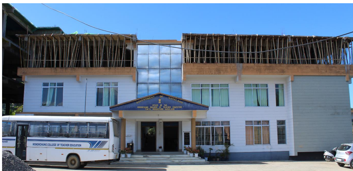
MCTE Administrative & Academic (Under Construction) Building
